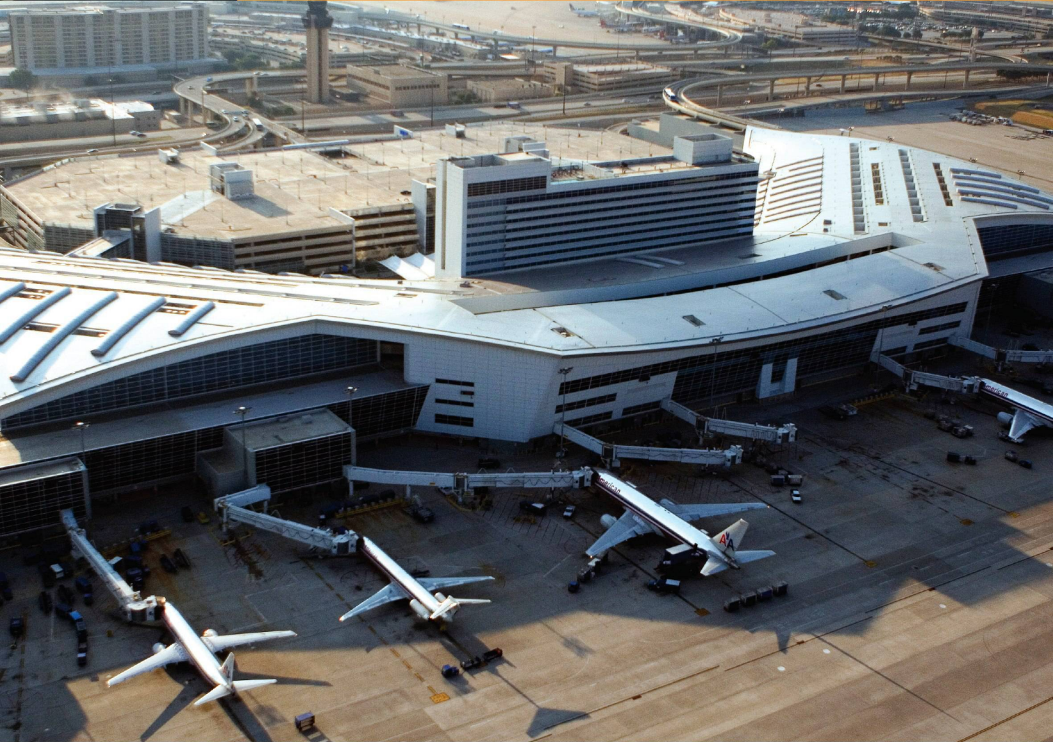
photo courtesy of DFW International Airport
